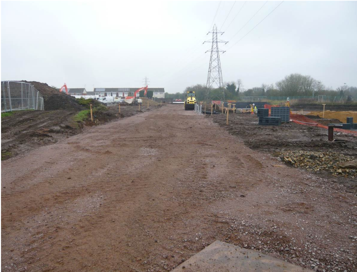
Road Sub-base Layer
