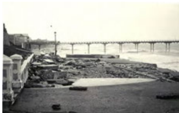
Figure 42: View towards the Pier showing flood damage to the promenade, January 1953
