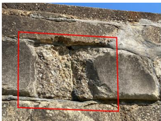
Blockwork seawall repair
