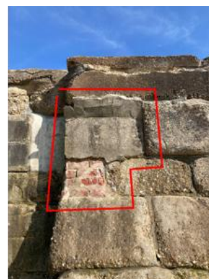
Blockwork seawall repair
