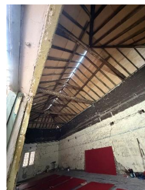
Roof works to the Red Barn
