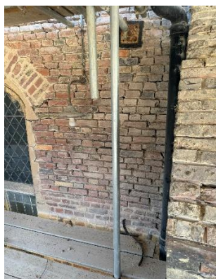
Guildhall Masonry Repointing
