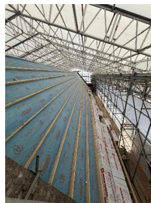
Guildhall Roof Works
