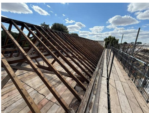
Roofworks to the Old Warehouse
