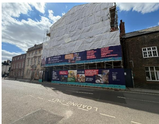
New Signage Installed
