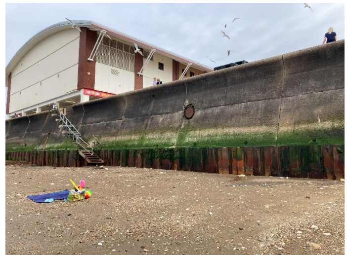
Seawall Section G
