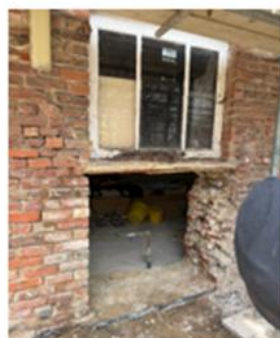
New doorways being installed
