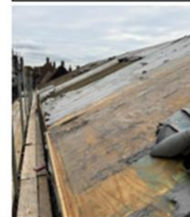
White Barn Roof being stripped
