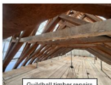
Guildhall timber repairs
