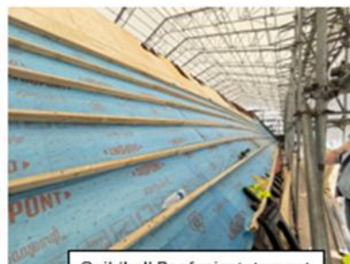
Guildhall Roof reinstatement
