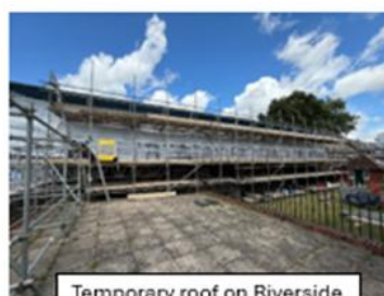
Temporary roof on Riverside
